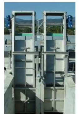
Mechanical screen with rakes of bar vertical way and linear in motion. They are installed in the wastewater channel with angle of  $70 - 75^{\circ}$ . The equipment consists of screen, motor reducer, base frame, chain mechanism, rake and rake cleaning system. The motion is conveyed to the rakes with the help of the chain mechanism. Number of the rakes depends on to the depth of channel and in the consequence of the length of the screen.
